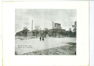
Tramway shed / depot © Publishing house "Minalo"
