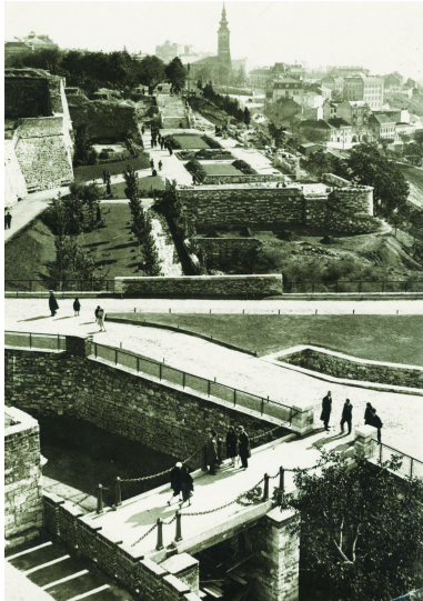
View of Kalemegdan Park © The Museum of Applied Art
