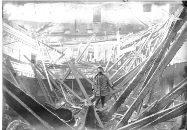
Fireman on the collapsed roof of the 'Kasina' cinema © Photoarchive Borba
