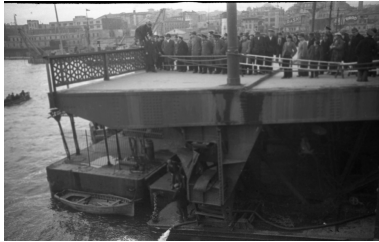
Line-up on the Atatürk Bridge construction site © Yapı Kredi bank
