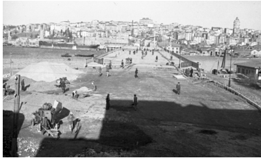
Visiting Atatürk Bridge under construction © Yapı Kredi bank
