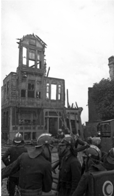
Firemen in front of a burnt-out wooden house in Sultanahmet © Yapı Kredi bank
